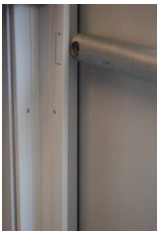
Bend fixing strip and place in corner with wider section on the door side.
