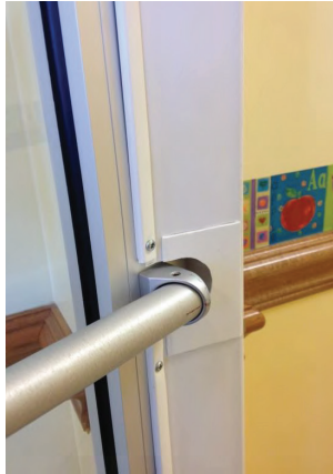
Fixing Strip and Accordion must be notched. Note: screw placement and reinforcement.
